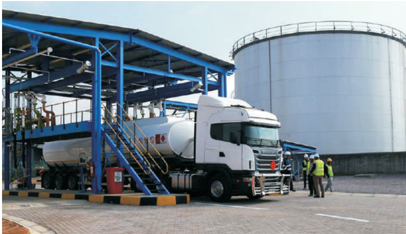
Tank farm in Nigeria
